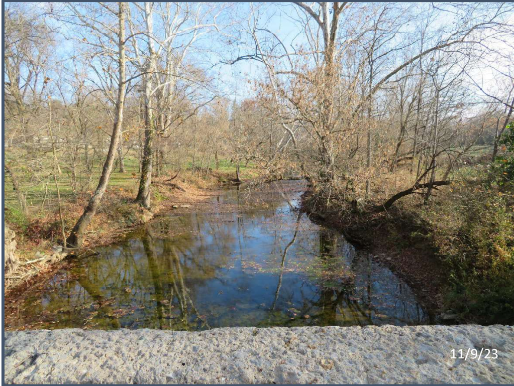
3) Looking east (upstream) at Leatherwood Creek from east side of the center of bridge 172
