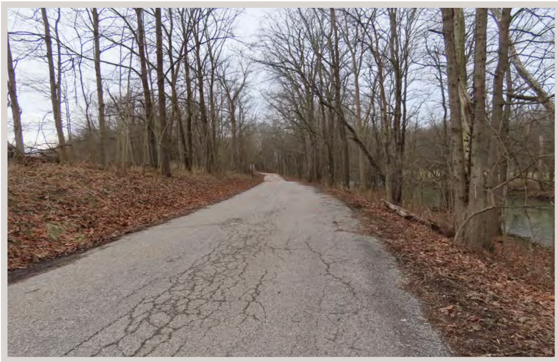
Photo 11: Looking southwest along Cement Plant Road towards the southern project terminus.
