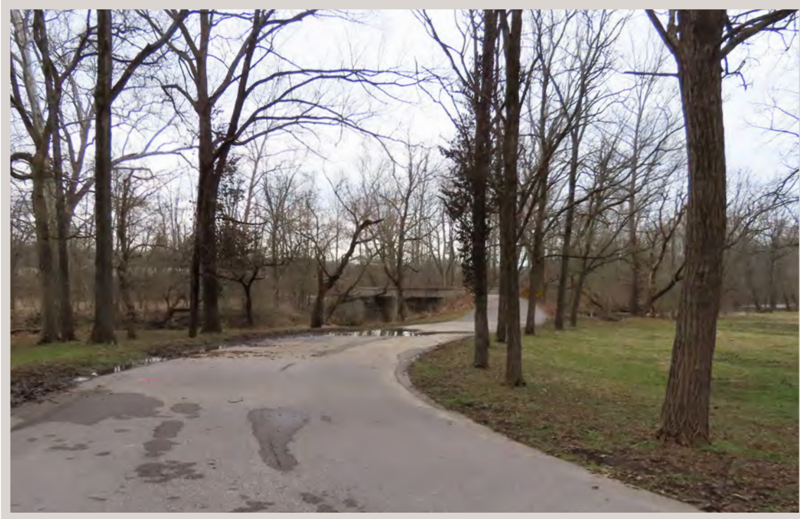
Photo 3: Looking southeast along Cement Plant Road towards Lawrence County Bridge 172.
