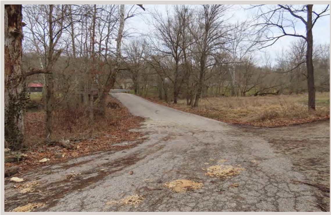
Photo 9: Looking northwest along Cement Plant Road towards Lawrence County Bridge 172.
