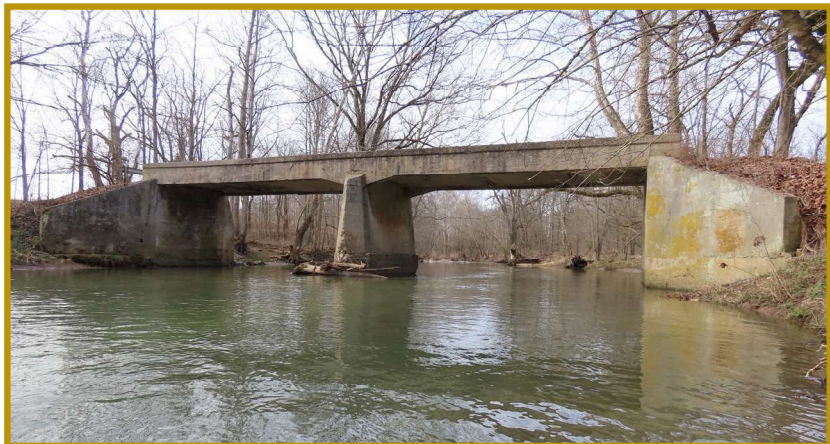
Photo 1: North elevation of Lawrence County Bridge 172.
