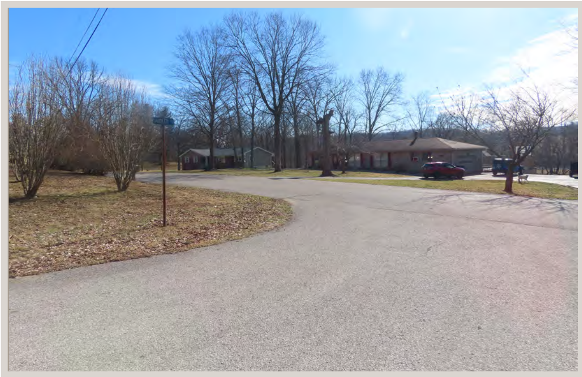
Photo 5: Looking southeast along Saddler Drive from Saddler Court.
