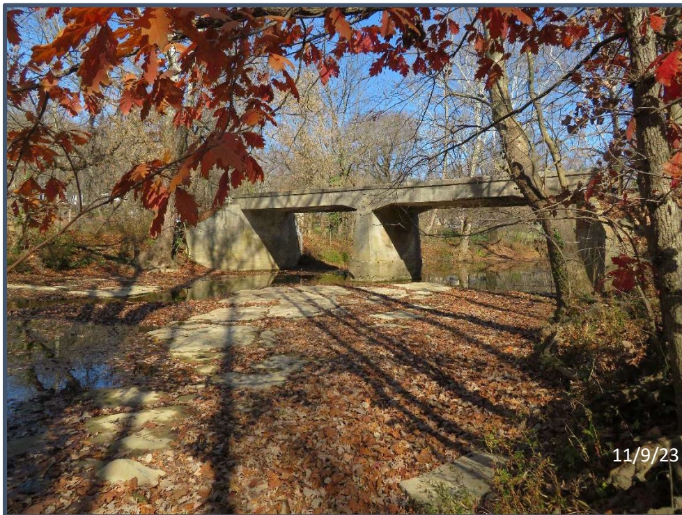
2) Looking east (upstream) at Leatherwood Creek passing beneath Bridge 172
