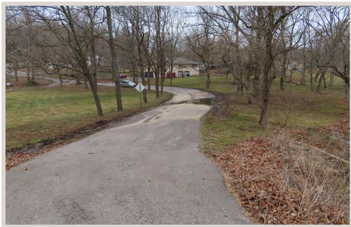
Photo 4: Looking northeast from Lawrence County Bridge 172.
