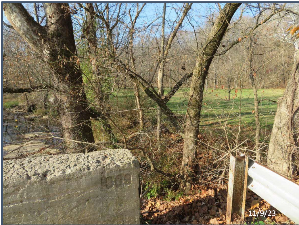
6) Looking northwest from Bridge 172 at the northwest quadrant of the bridge
