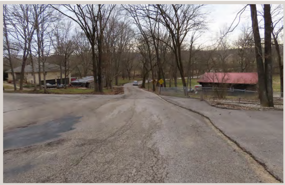
Photo 2: Looking southeast along Cement Plant Road from Saddler Drive, towards Lawrence County Bridge 172.
