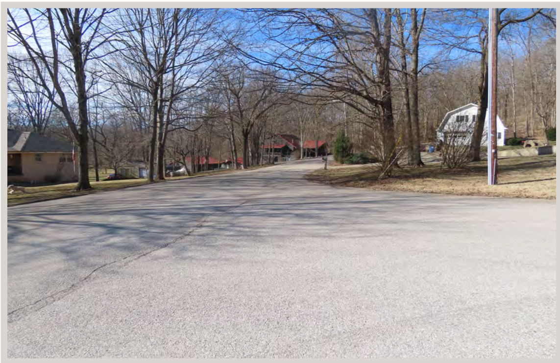
Photo 6: Looking west along Saddler Drive towards Cement Plant Road.
