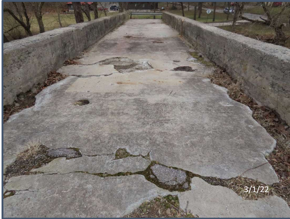
1) Overview of project location, looking north along Cement Plant Road
