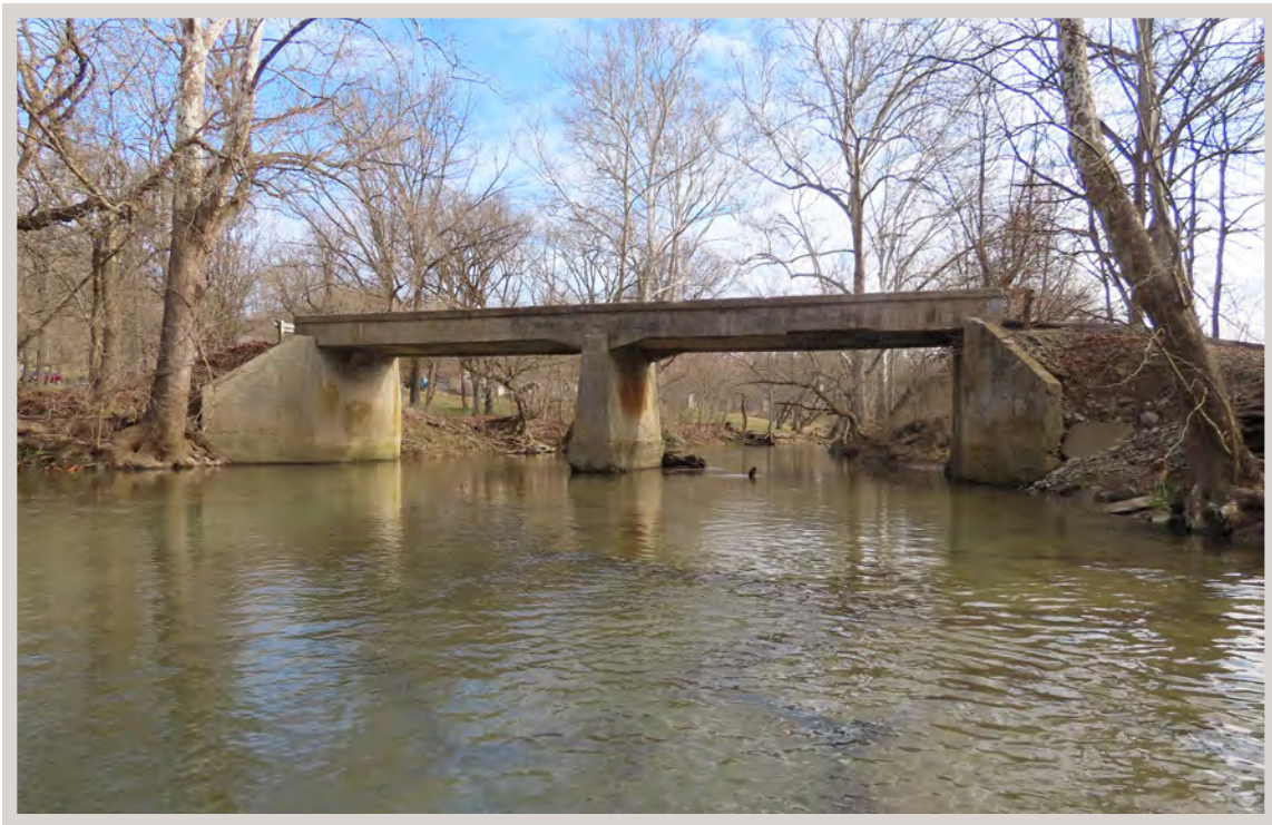
Photo 12: Looking north at the south elevation of Lawrence County Bridge 172.
